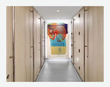
unique 3-part aluminum headrail system, the full height stalls offered maximum privacy to employees with 20mm floor and ceiling clearances.
